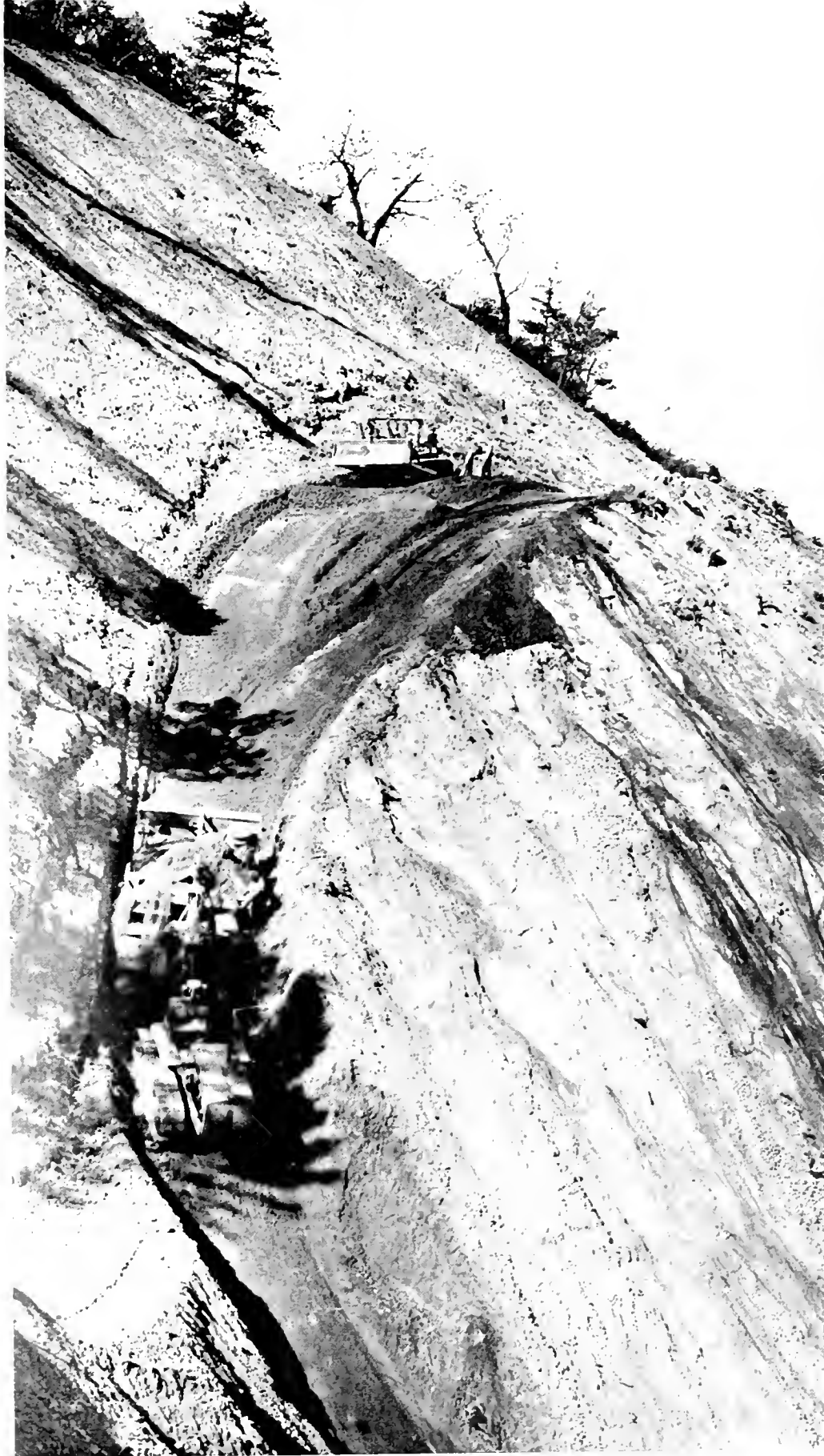
Grading down steep mountainside for Antler Bridge approach
